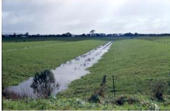
**Figure4. Hump and hollow drains are suitable for areas with a high water table.**
