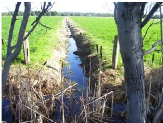
**Figure 1. Open arterial ditches lower the water table and remove water from paddocks.**
